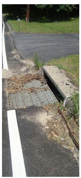
Pavement overlay creates large drops at storm drain and requires pavement milling to reduce hazards to bicyclists
